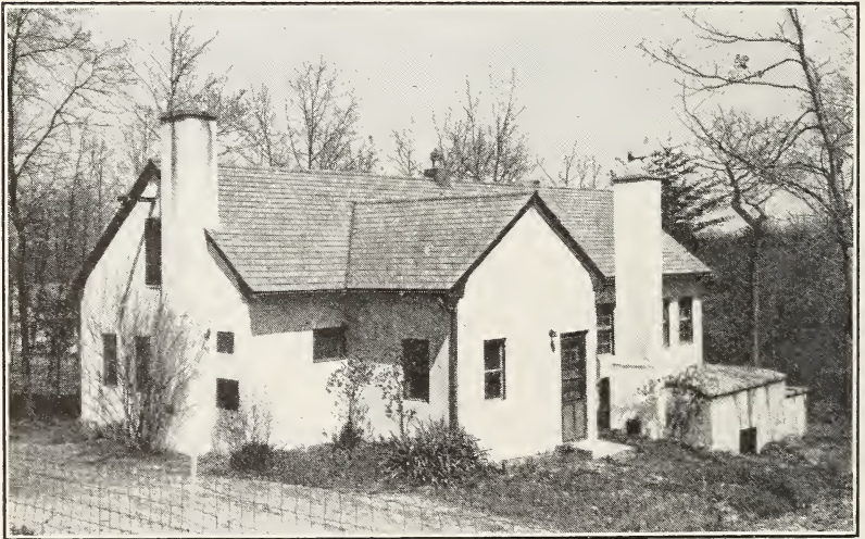
FIGURE 23.—The coccidiosis building on the Zoological Division's section of the poultry farm. This building serves as an isolation unit for all experimental work with coccidiosis of poultry. The incinerator shown at right is connected with the main building by means of chutes and is used for burning all litter and other material from the experimental pens.
